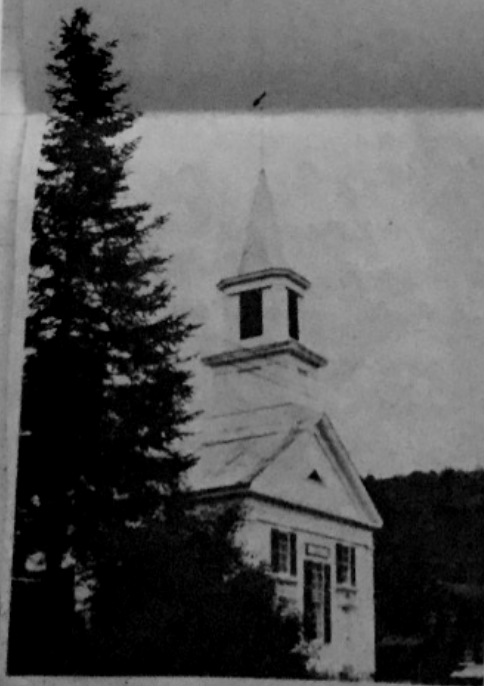
Look closely The Steeple of the West Fairlee Center Church is visibly leaning. Unless repairs are made soon, the historical church will lose its spire altogether.
